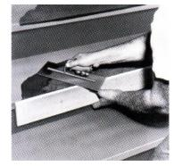
American Stair Treads recommends using Tapcon Screws to fasten down metal stair treads. This is the most popular method of securing the treads. Tapcon screws offer many advantages such as: No layout or hole-spotting required, Fast & easy installation, Removable, Use with masonry drill bit for maximum holding power. Tapcon screws have a recommended embedment of 1" to 1-3/4".
